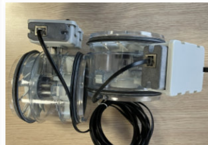
4/ The 2 e-VAV are now connected in master/slave mode
